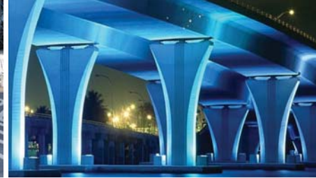
LIGHT COLUMNS & CEILINGS
