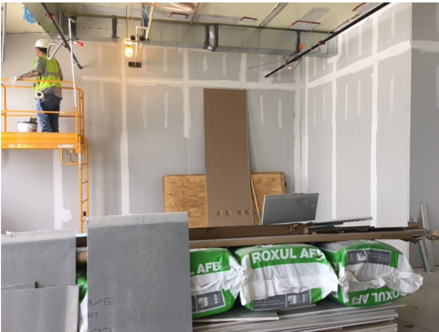
Drywall installed in classrooms
