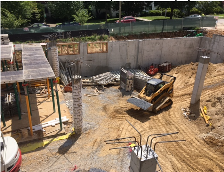
Concrete work in the cafeteria
