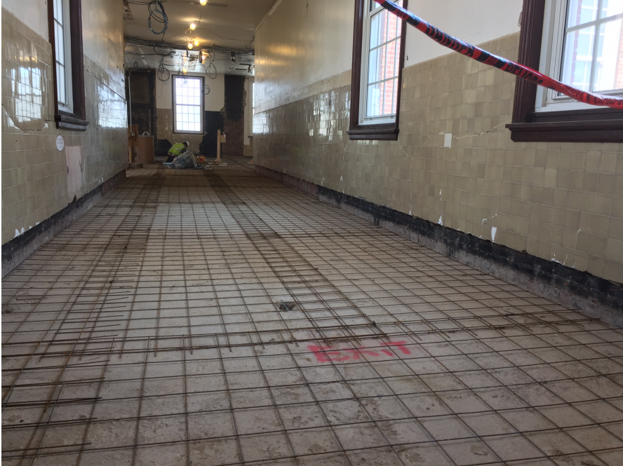
Preparing to pour the concrete topping slab to level the floors
