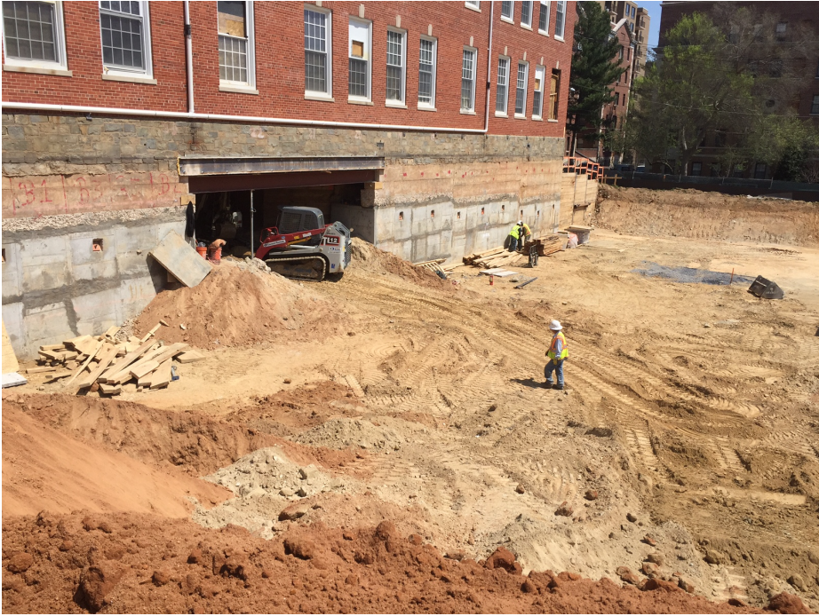
Future site of the cafeteria
