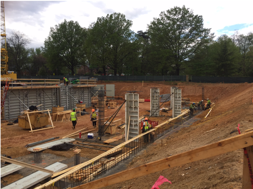
Concrete work for the garage and basement
