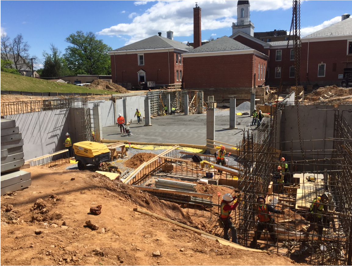
Concrete foundation work for the garage
