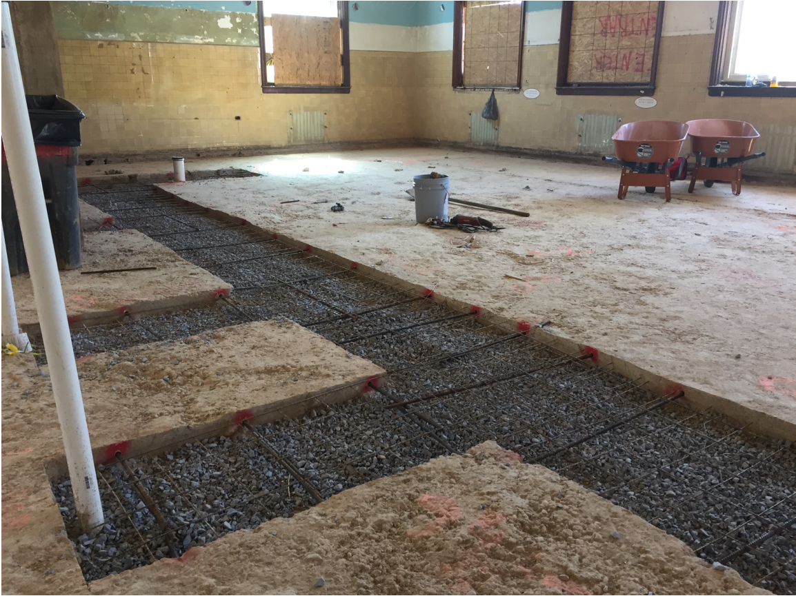
Preparation for pouring the concrete topping slab on the first floor
