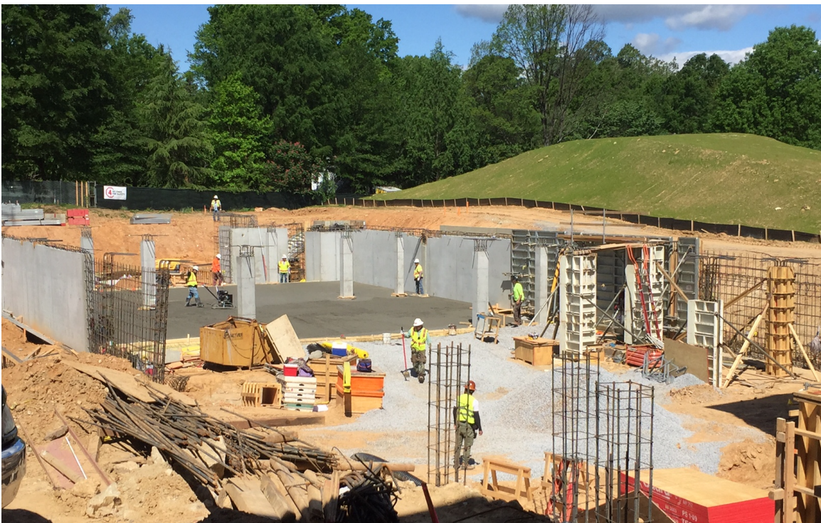
Concrete foundation work for the garage
