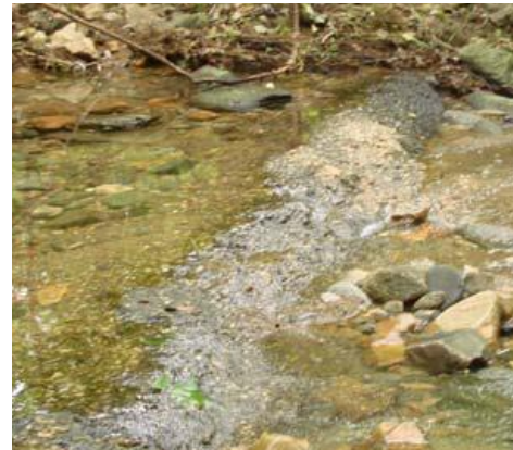
At-risk Sewer Pipe Crossing Stream
